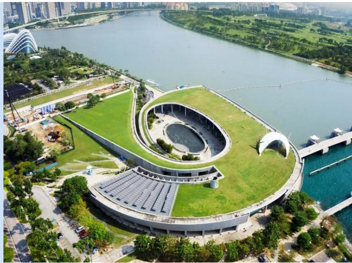
Gambar 2.38 Aerial View Marina Barrage (Sumber: Visitsingapore.com, 2025)
