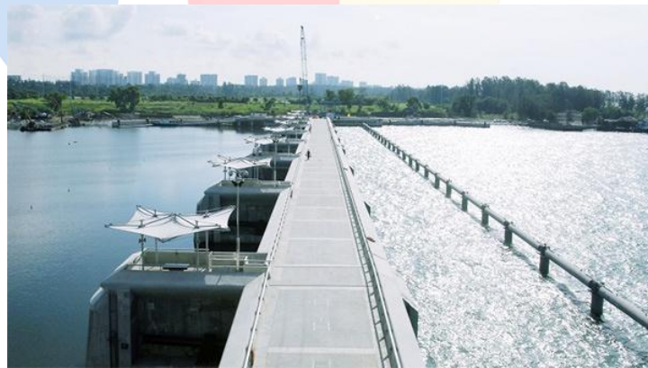
Gambar 2.42 Bendungan di Marina Barrage (Sumber: PUB Singapore's National Water Agency, 2025 )
