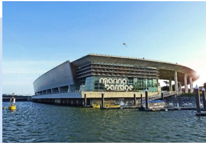
Gambar 2.37 Marina Barrage , Singapura (Sumber: PUB Singapore's National Water Agency, 2025)
