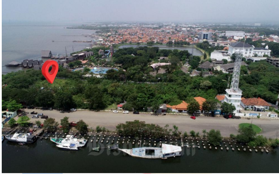
Gambar 5.5 Aerial View eksisting tapak.
