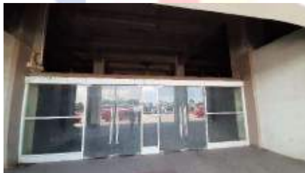
Gambar 4.54 Supermarket (on progress) di Terminal Terpadu Pulo Gebang Sumber: Dokumen Pribadi, 2020
