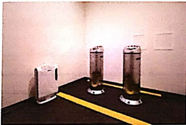
Figure 4.1.3 Hotel Facilities: Smoking Room (1 st Floor)
