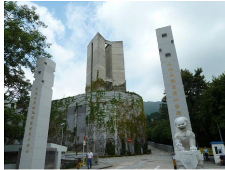
Gambar 2. 29 Entrance Diamond Hills Crematorium
