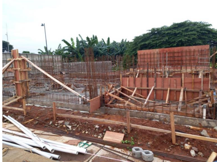
Gambar 4.2.2.2 Pengerjaan Water Features
